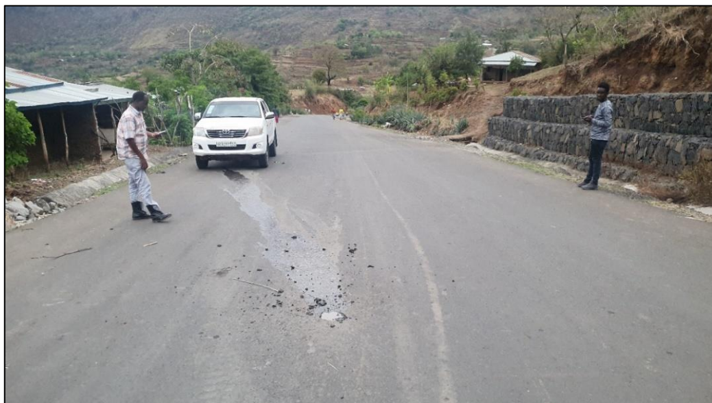
Figure 3-4: Pumping of water through new placed asphalt concrete road @ km 105+000
