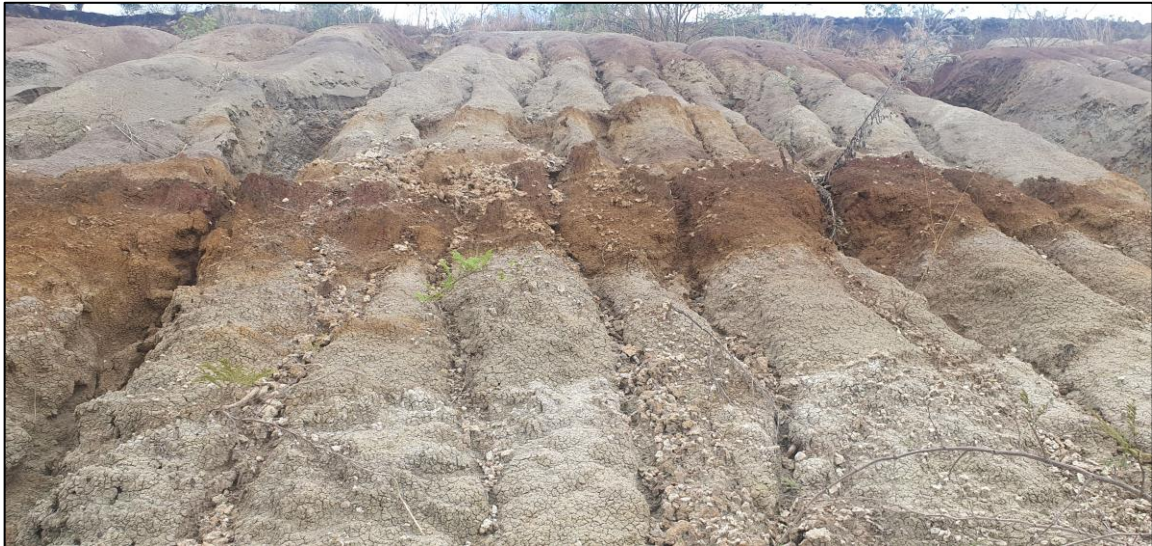
Figure 4-11: Formation of cracks, fissures, looseness and crumbliness of soils on the slope surface
