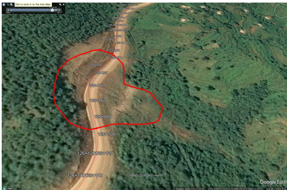
Figure 4-43: Google earth historical imagery dated October, 2014 at km 126+000 (LHS)
