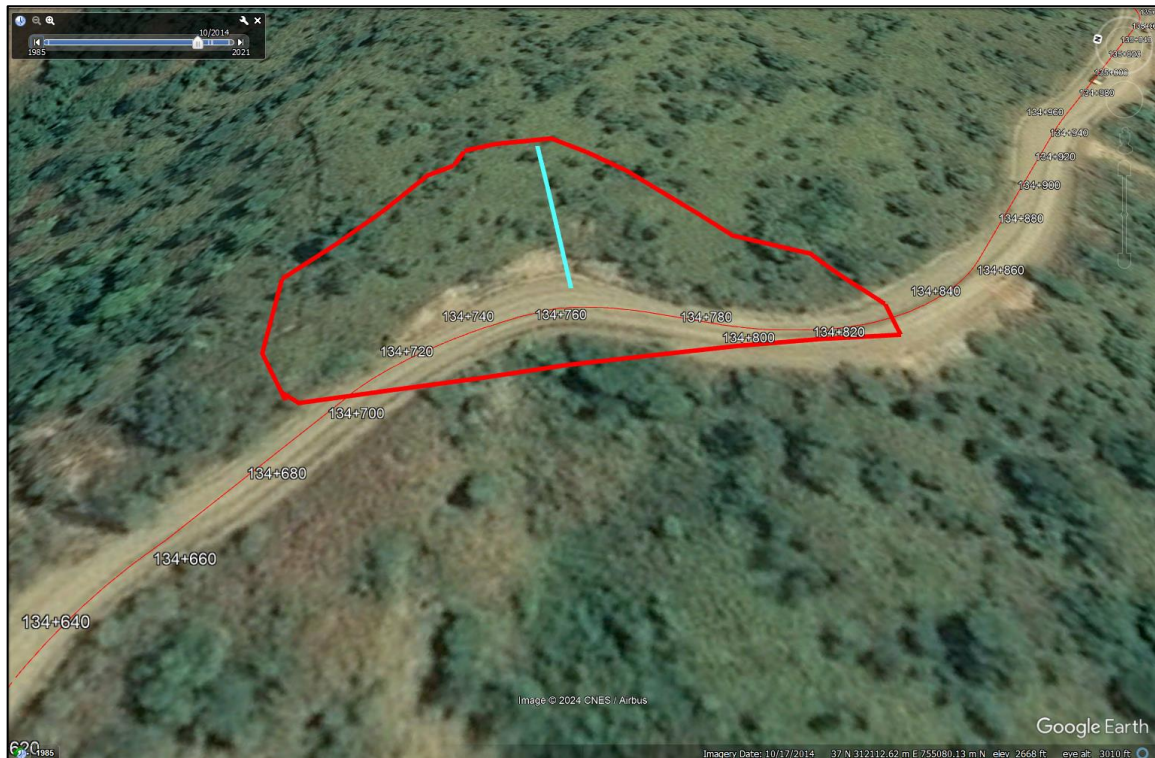
Figure 4-17: Google earth historical imagery dated October, 2014 @ km134+760 RHS
