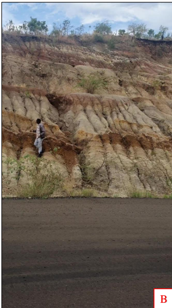
Figure 4-8: A & B) Formations of rills and gullies on the surface of slope C) Crack and fissures on the surface of slope soil
