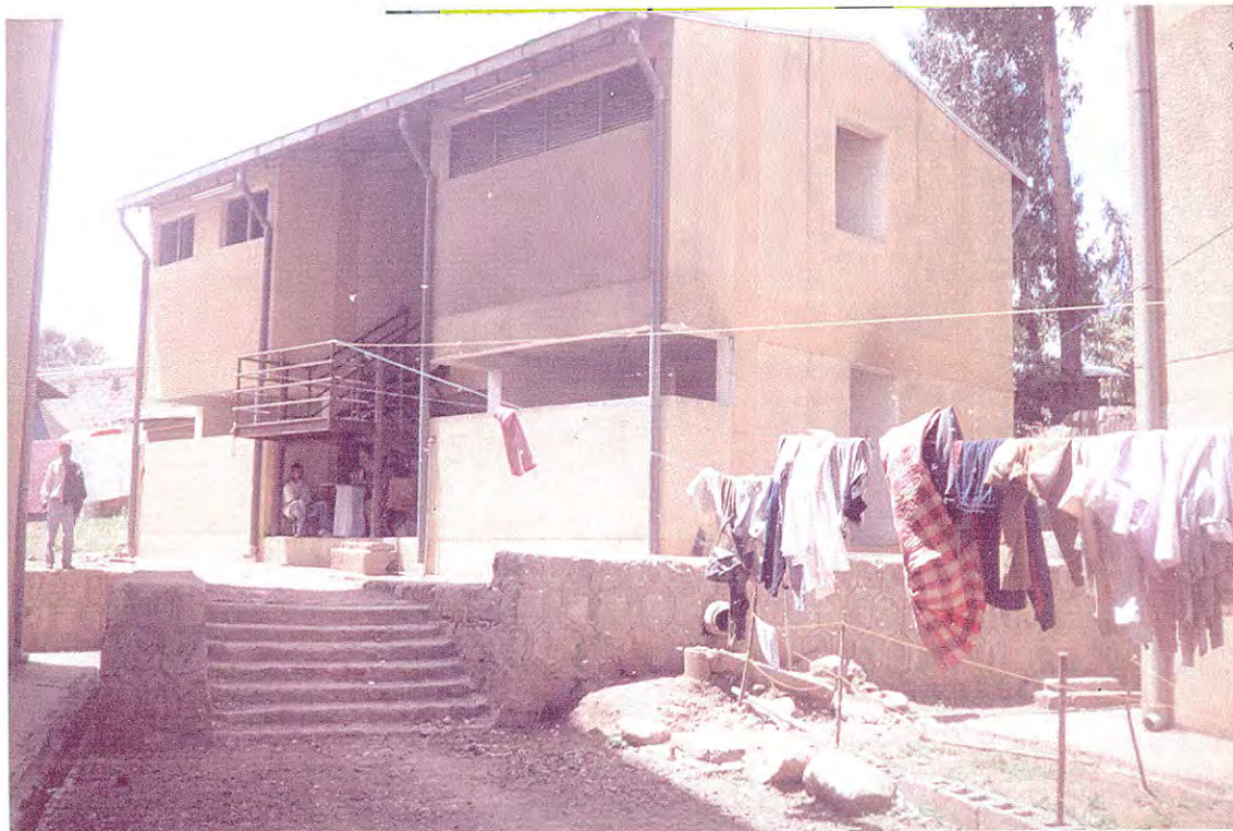
Figure 3.14: Communal house, occupied kitchen, place for washing cloths and slaughtering animals. Photo taken from Ras Desta site.
