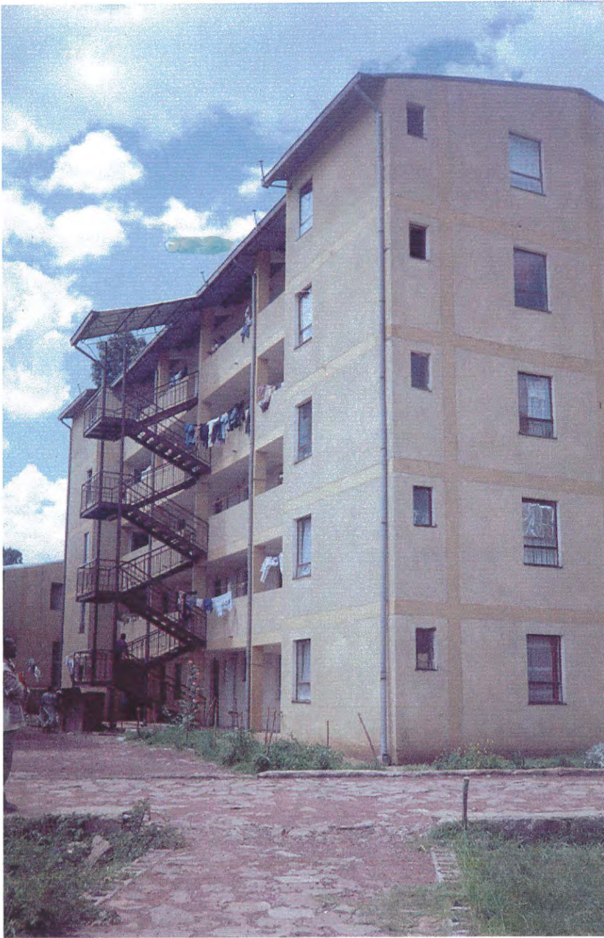
Figure 3.18: Stair case. Photo taken from Ras Desta site.
