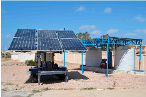
Figure 9: Semipermeable Membrane Reverse Osmosis (SPRO) desalination system [3]
