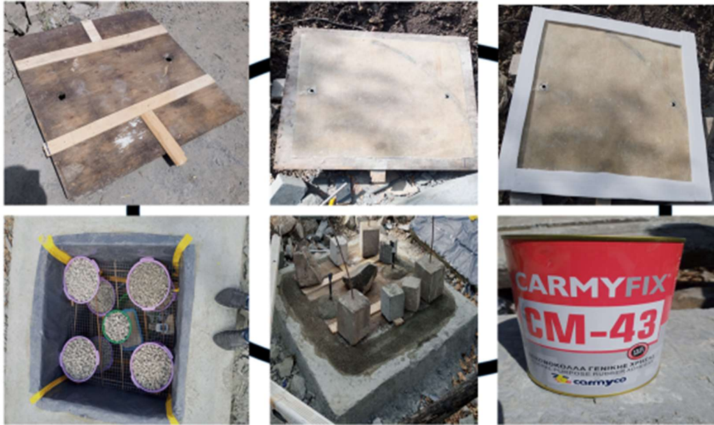
Chamber construction and testing cont.
