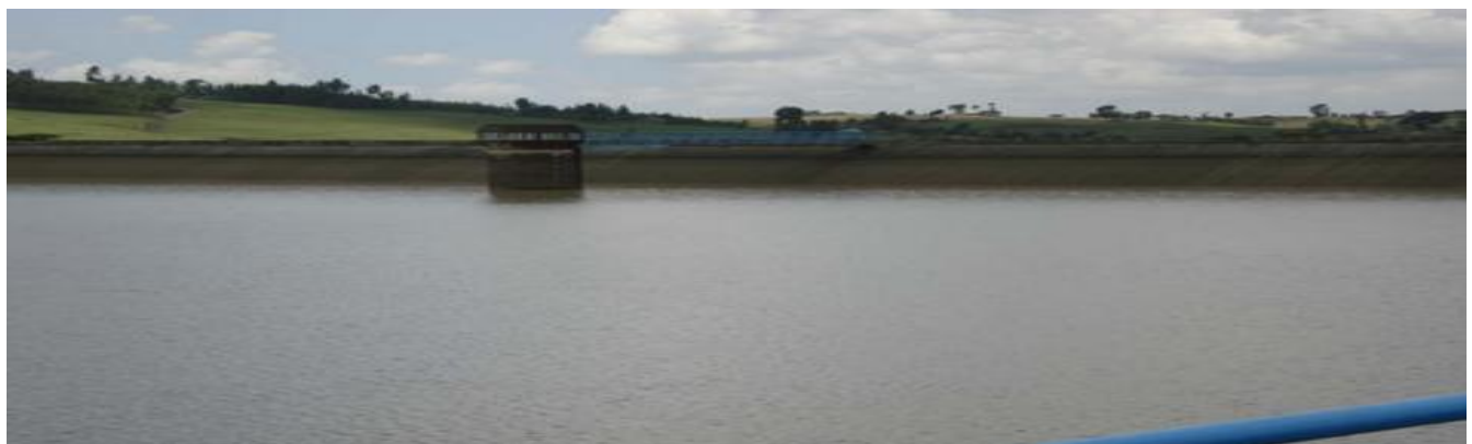
Legedadi Water Reservoir
