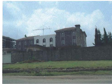
Figure 4.17 Algeria Embassy Chancery.
