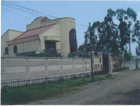
Figure 4.29 Neighboring Rented Residence
