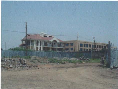
Figure 4.41 Office converted to Luxurious Residence
