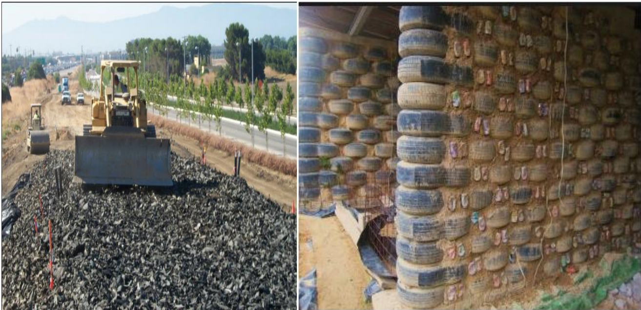
Figure 2.3: sample use of waste tire for road construction and building [24]
