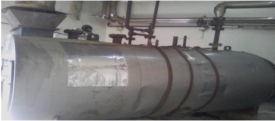
Figure 8. 4 Boiler surface of the factory
