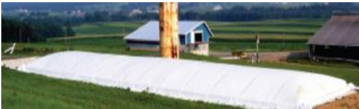
Figure 14- Plug Flow Digester on a Dairy Farm
