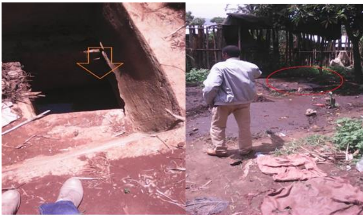
Figure 4.3: Outlet tank hole in to salary pit was blocked biogas plant in HT woreda (Source: field survey of 2018)
