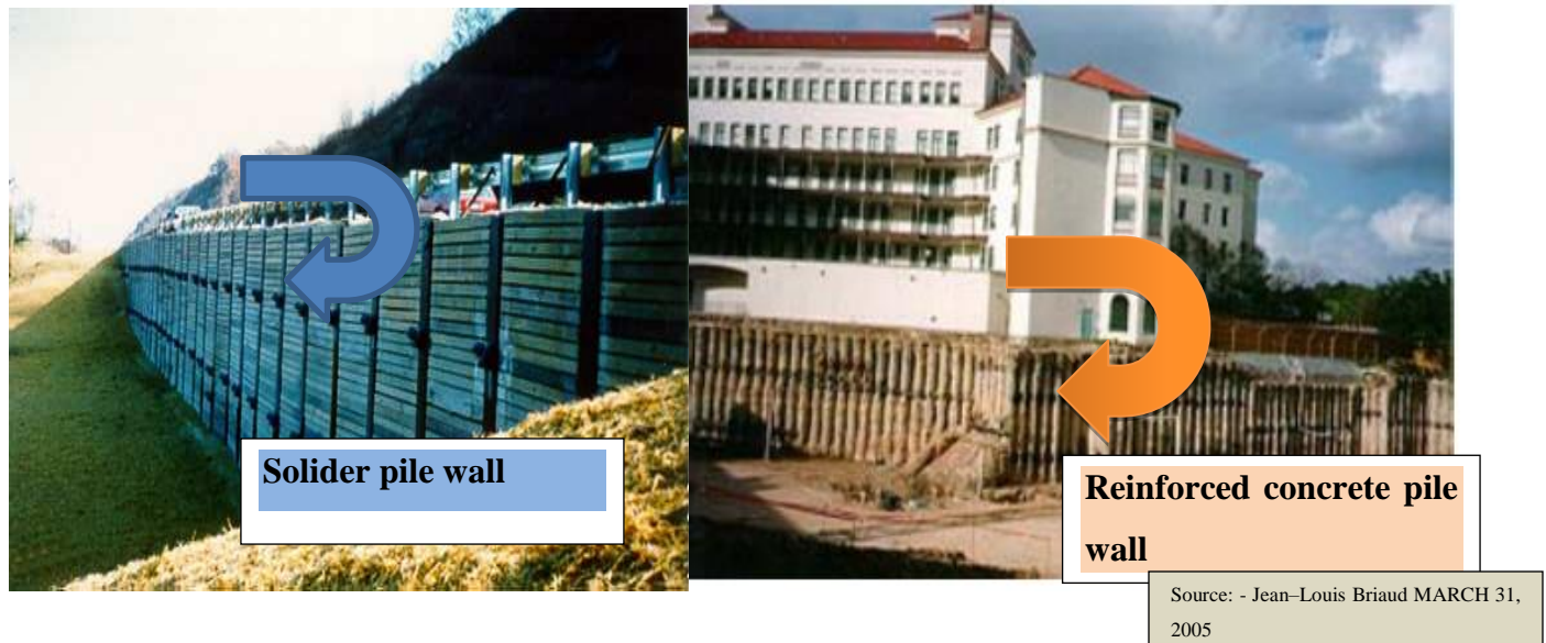
Figure 1: soldiers with timber lagging and reinforced concrete pile wall
