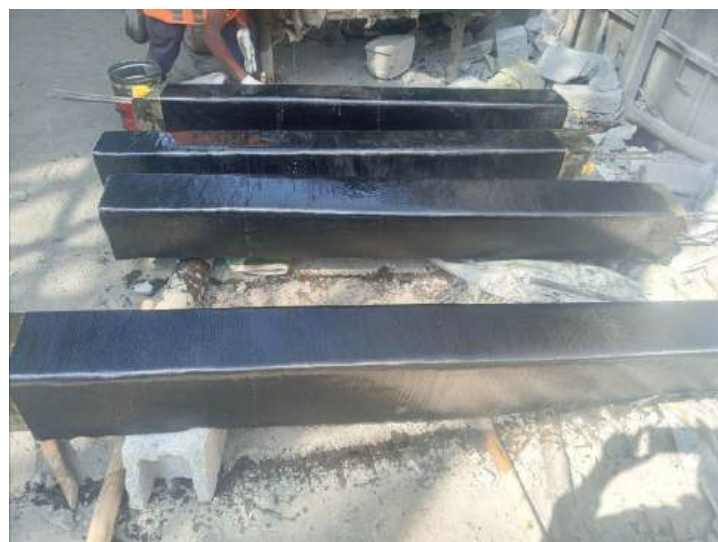
Figure 3.7: Wrapping of CFRP
