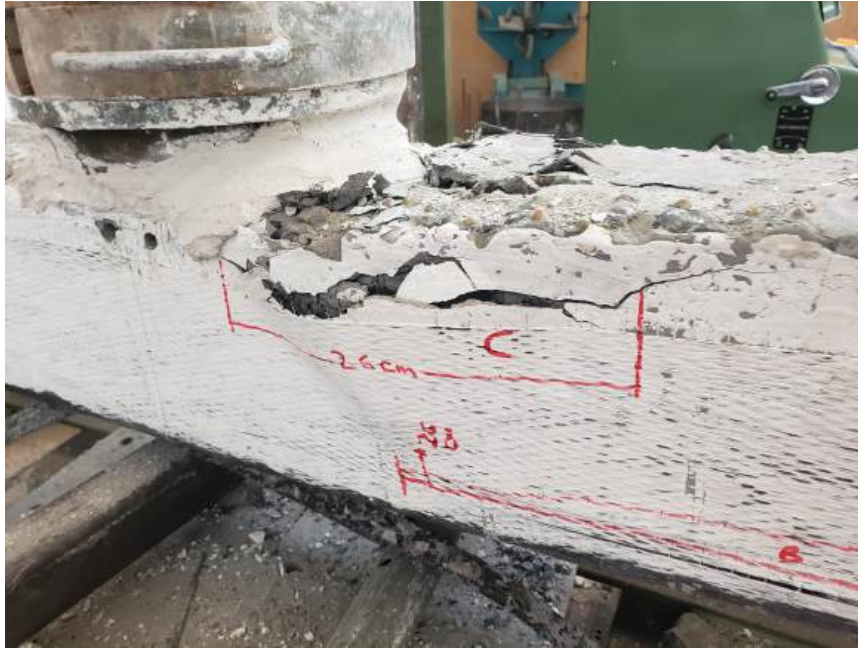
Figure A.6: Concrete Crushing and Spalling at top of the beam
