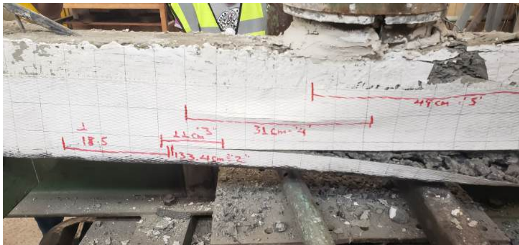
Figure A.10: G2B-12 Right Side CFRP Tear & Delamination
