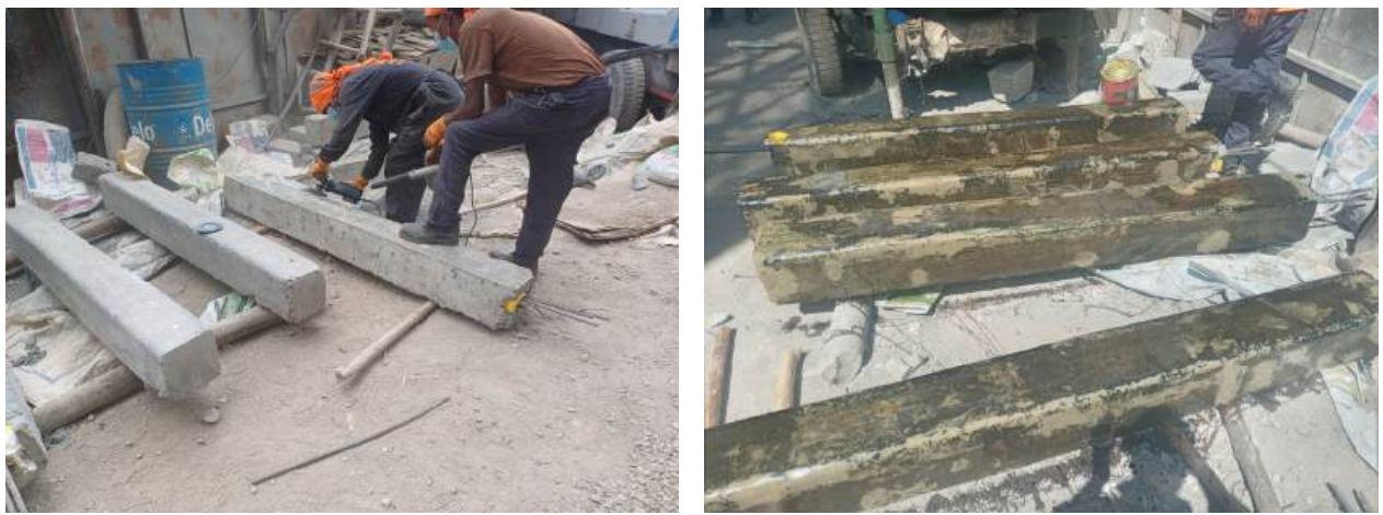
Figure 3.6: Polishing & Primer Application (left to right)
