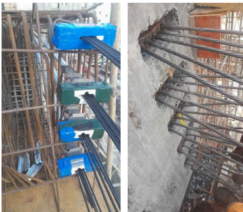
Figure 2.1: Post Tensioned Beam with Bonded Tendons
