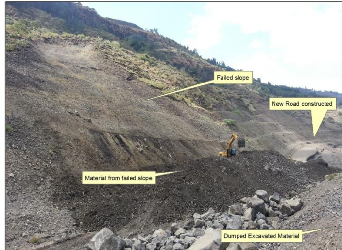
Plate 7.1 Photo showing the excavation activities taking place during field work
