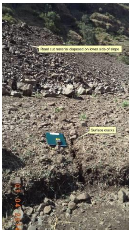
Plate 6.20 Photo showing disposal material placed at lower side of the road cut slope
