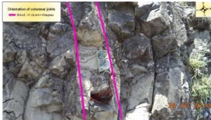
Fig 4.8b Columnar joints tilted in N - W directions
