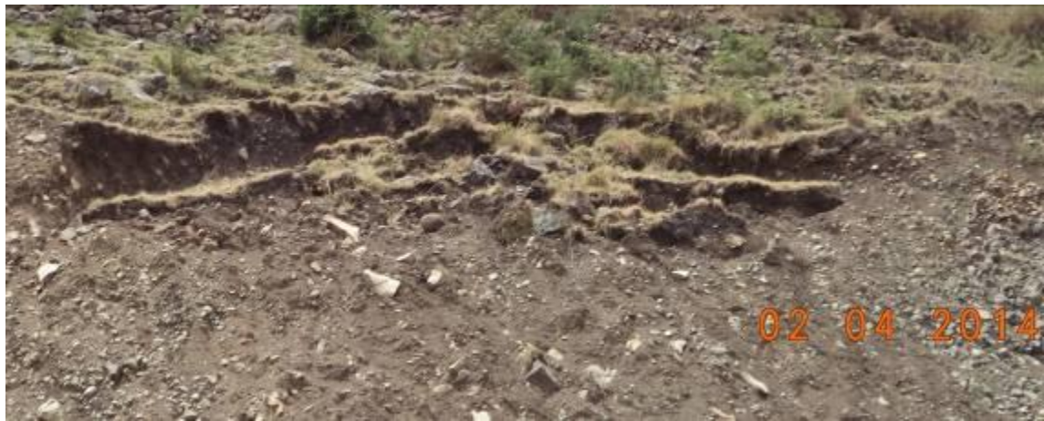
Plate 6.23 Soil slide triggered by slope cutting activities during road construction
