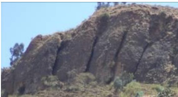
Plate 6.15 Photo showing rocks with open sub-vertical joints on cliff susceptible to fall/topple
