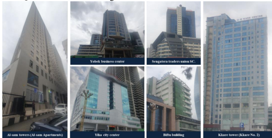
Figure 13: comparable High-rise commercial buildings in the study area Source: Author's photograph
