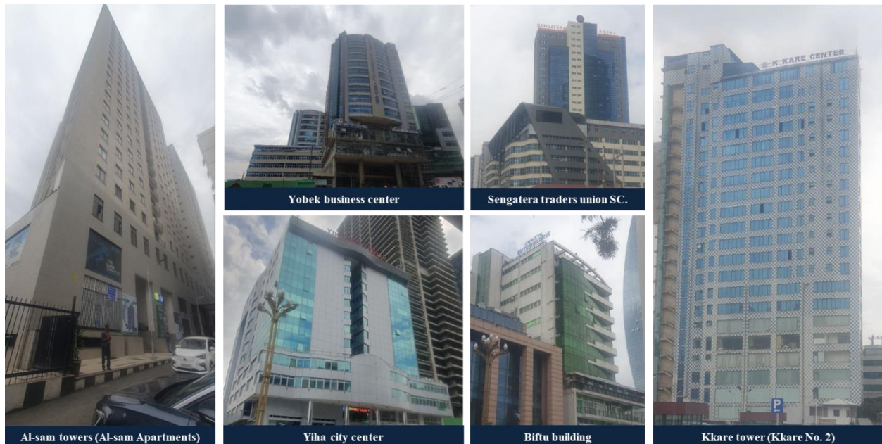
Figure 10: High-rise commercial buildings in the study area
