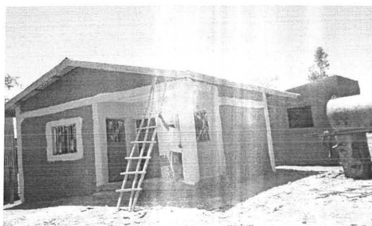
Under construction public veterinary clinic (Ude)
