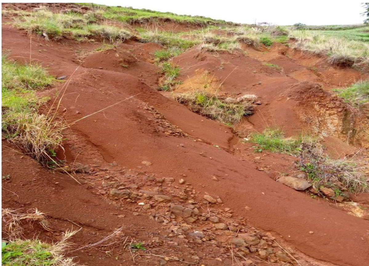
Figure 2. 1. The photo was taken from Gully land in Dega Damot District
