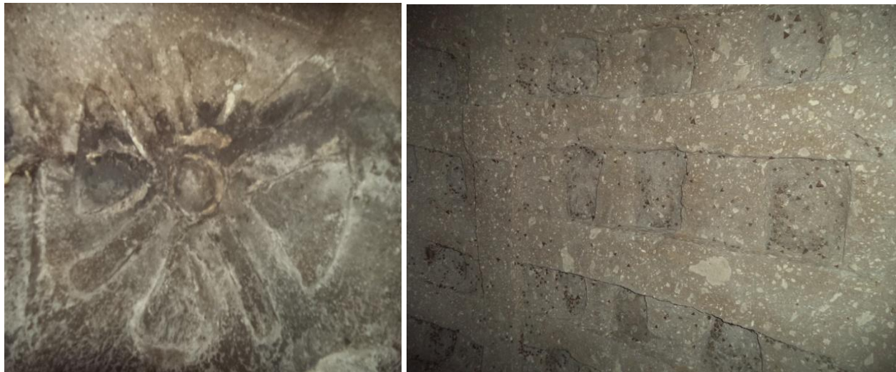
Figure 4.26 (left) Geometrical features on the nave's roof, Tefu Meskele Eyesus
