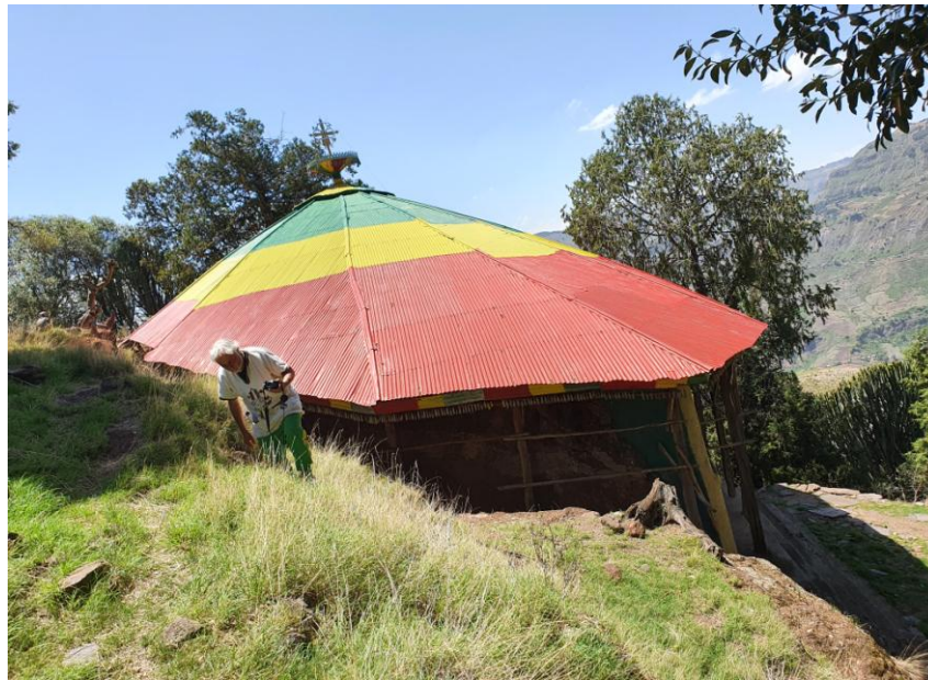
Figure 4.6 Mesenna Medhane Alem, sheltered with iron sheets
