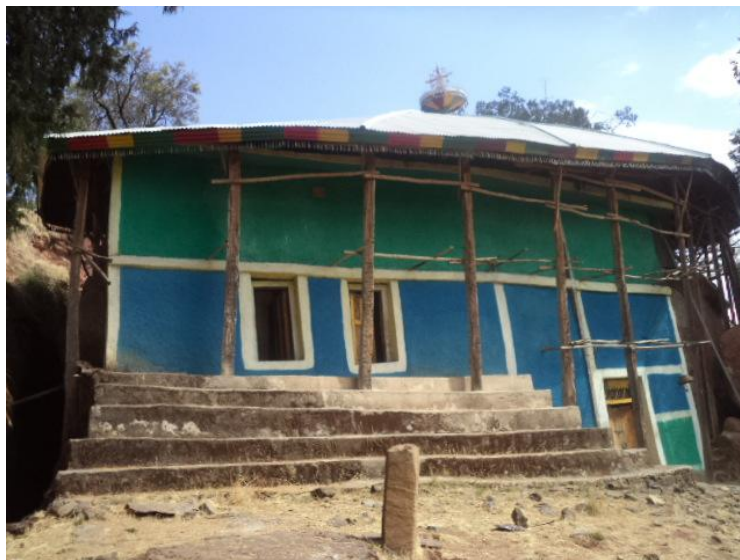
Figure 4.41 The repaired part of the frontal façade of Mesenna Medhane Alem
