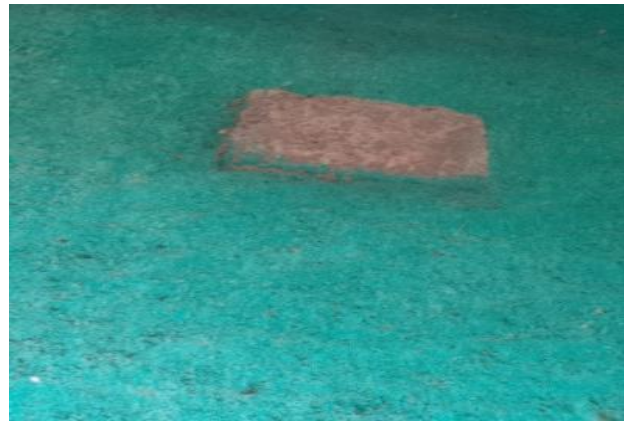
Figure 4.47: Bad repairing work made at Nazugn Mariam rock-hewn church
