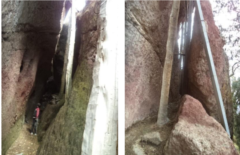
Figure 4.7 (left) Northern side of the trench of Mesenna Medhane Alem Figure 4.8 (right) Eastern end of the trench of Mesenna Medhane Alem
