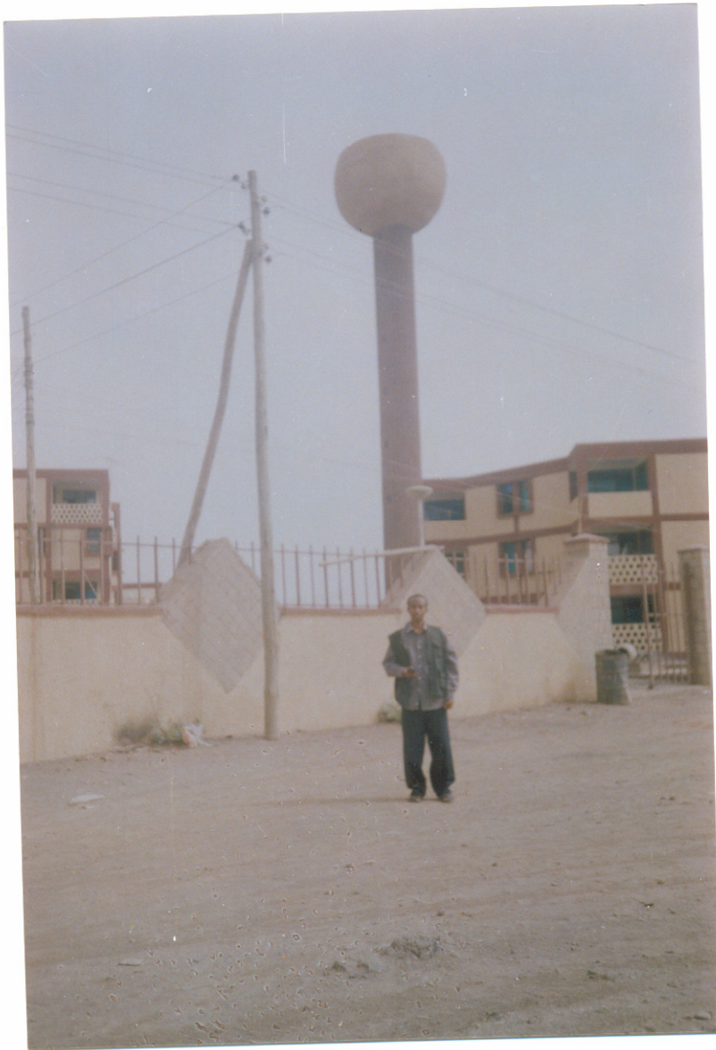
Fig. 6.2 A water tower in semera, vulnerable to earthquake hazard due to its height and narrowness.
