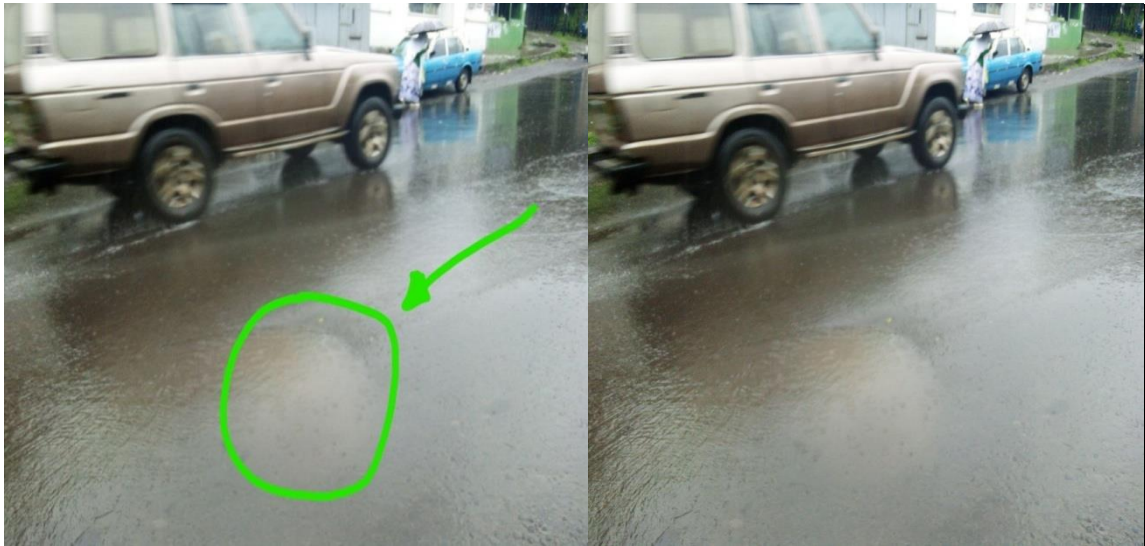
Figure 3: 13 Photos of Inflow on the existing sewer network
