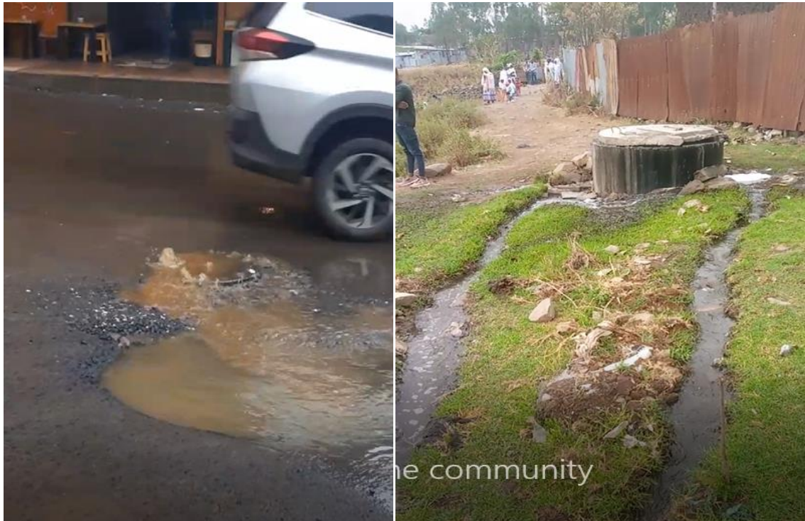
Figure 3: 10 Photos of overflow on the existing sewer network
