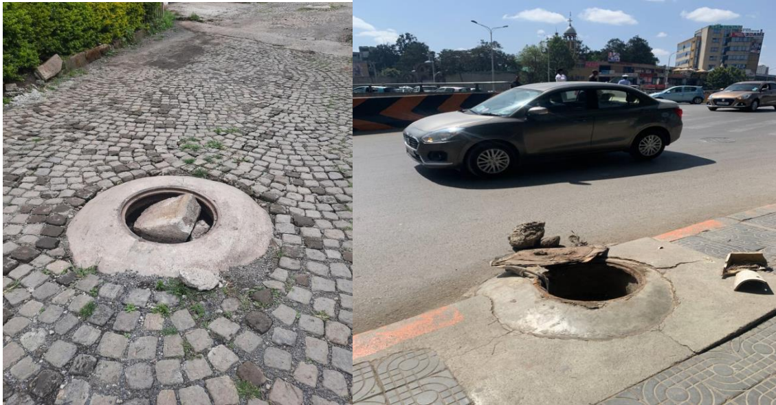
Figure 3: 11 Photos of open manholes on the existing sewer network
