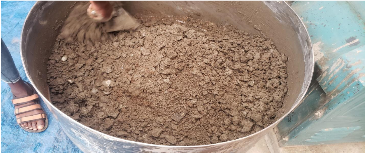
Pictures taken while mixing concrete
