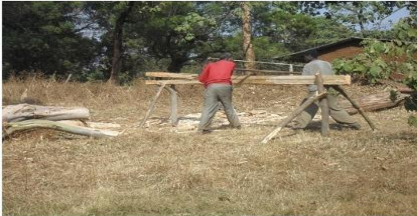
Figure 8. 16: Cutting and Preparing Construction Poles
