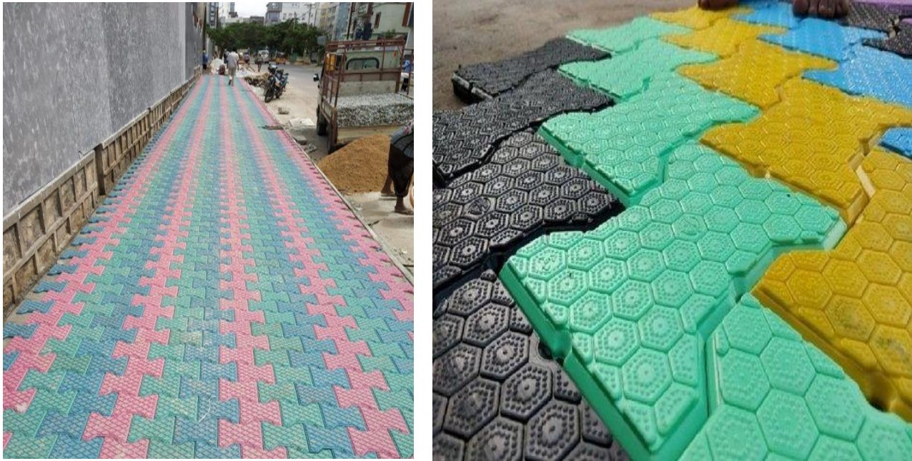
Figure 2.4 Plastic stabilized Pavement bricks in India
