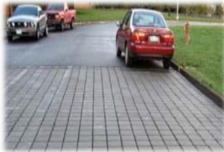
Figure 2.6: Permeable Pavement (source: [4])
