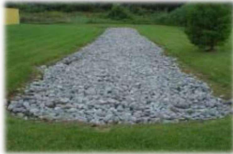
Figure 2.5: Infiltration Trenches (source: [4])
