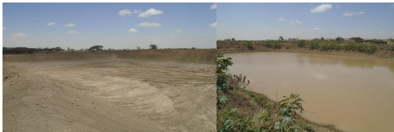
Environment situation before and after intervention
