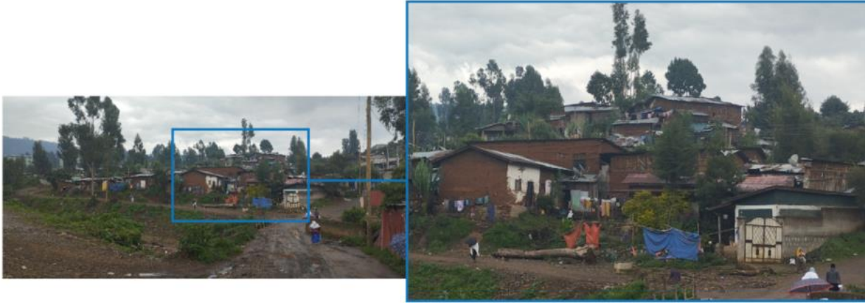
Figure 32-Earthen construction highlights around Qechenie area. Photo by author, [July, 2024].
