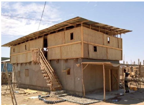
Figure 7- A building constructed using stabilized earth as a wall. Source; Kiessling, D(2017) .
