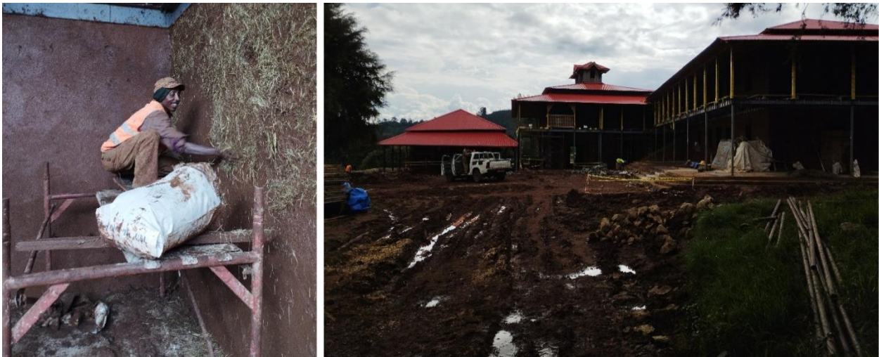
Figure 35-Ato Angasso involving in the Abba Jifar palace conservation and reconstruction project. Photo by author, [July, 2024].
