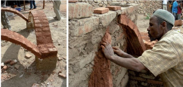
Figure 70- Earthen masonry vaulting. Source Building Ethiopia.
