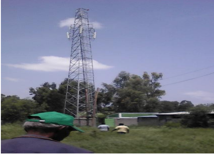
Figure 1: Mobile base station in the study area
