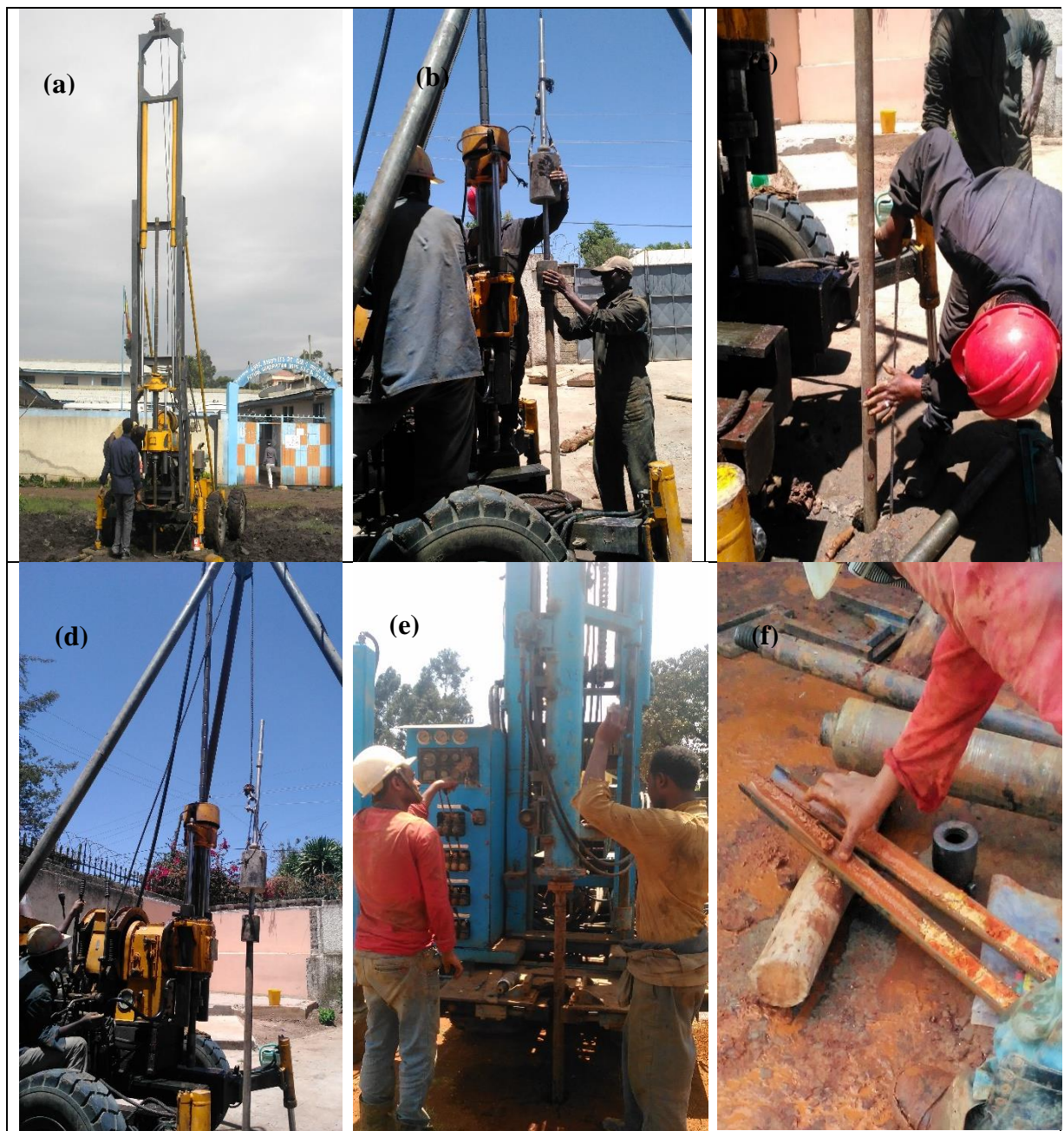
Plate 4.4 SPT test procedures: (a) drilled at target depth (b) assembled SPT Equipment (c) put marks on the rod three (d)&(e) conducting the test (f) Handling the samples.
