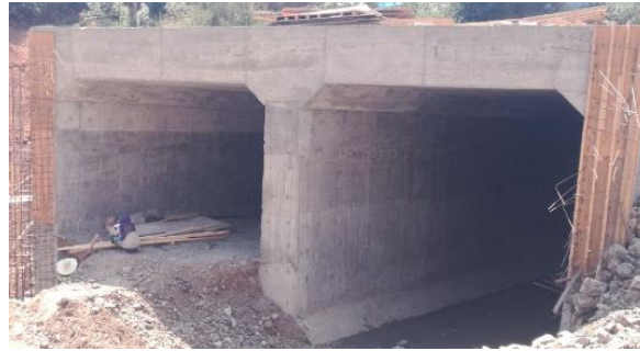
Figure 2-2 Cast in situ box culvert
