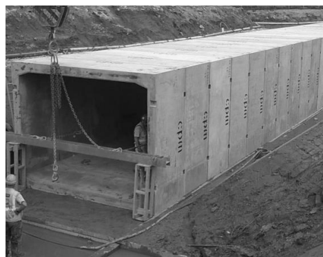
Figure 2-3 Precast box culvert [24]
