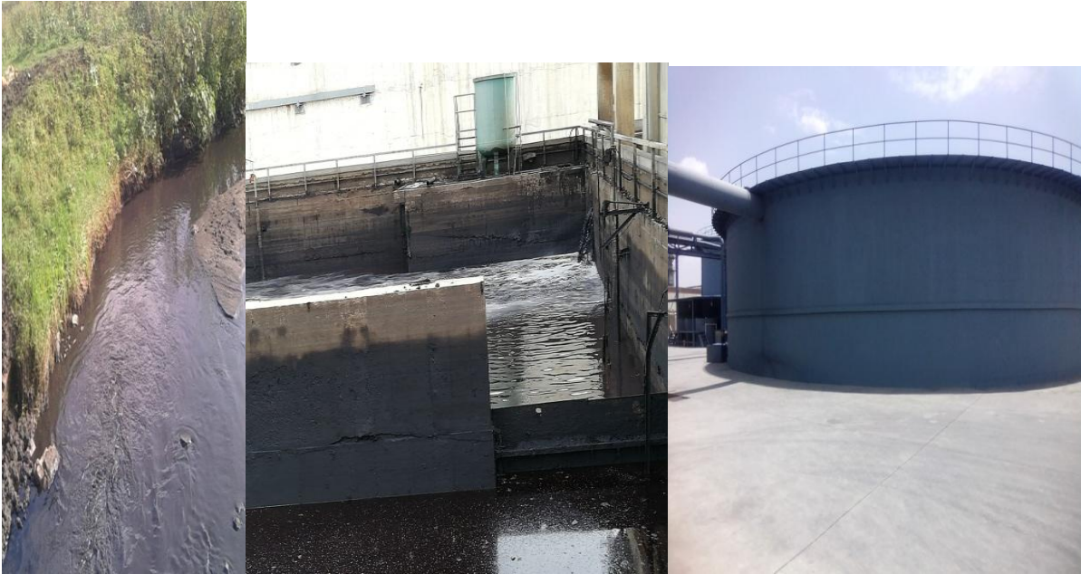
Figure 4.5: the communal treatment plant
