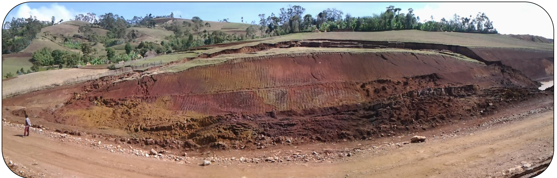
Figure 4.22: Front view of the slide and block movement of the slide mass
