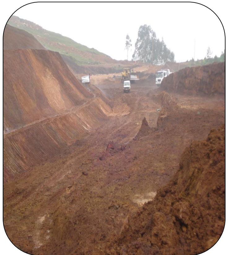
Figure 4.15: Common Excavation work on progress
