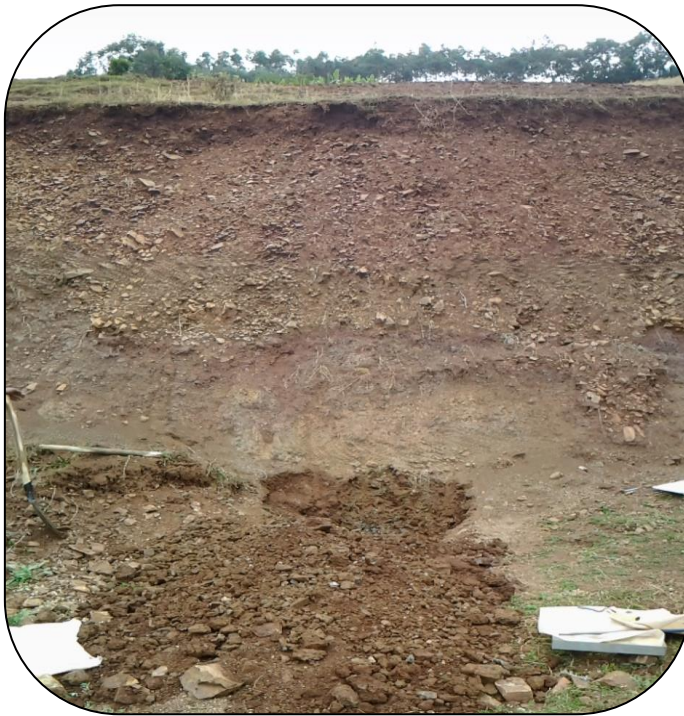
Figure 4.8: Granular exposed part of the slide plane material
