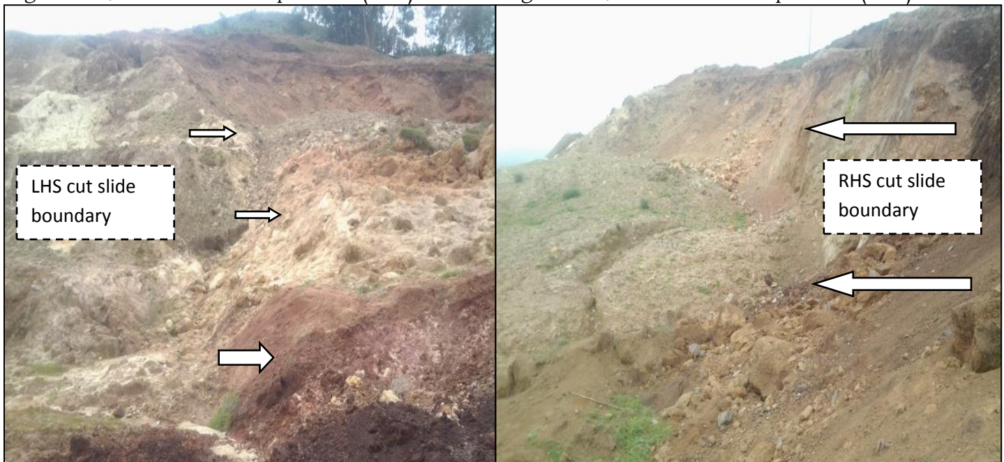
Figure 4.29: LHS view of cut slope failure (slide)
