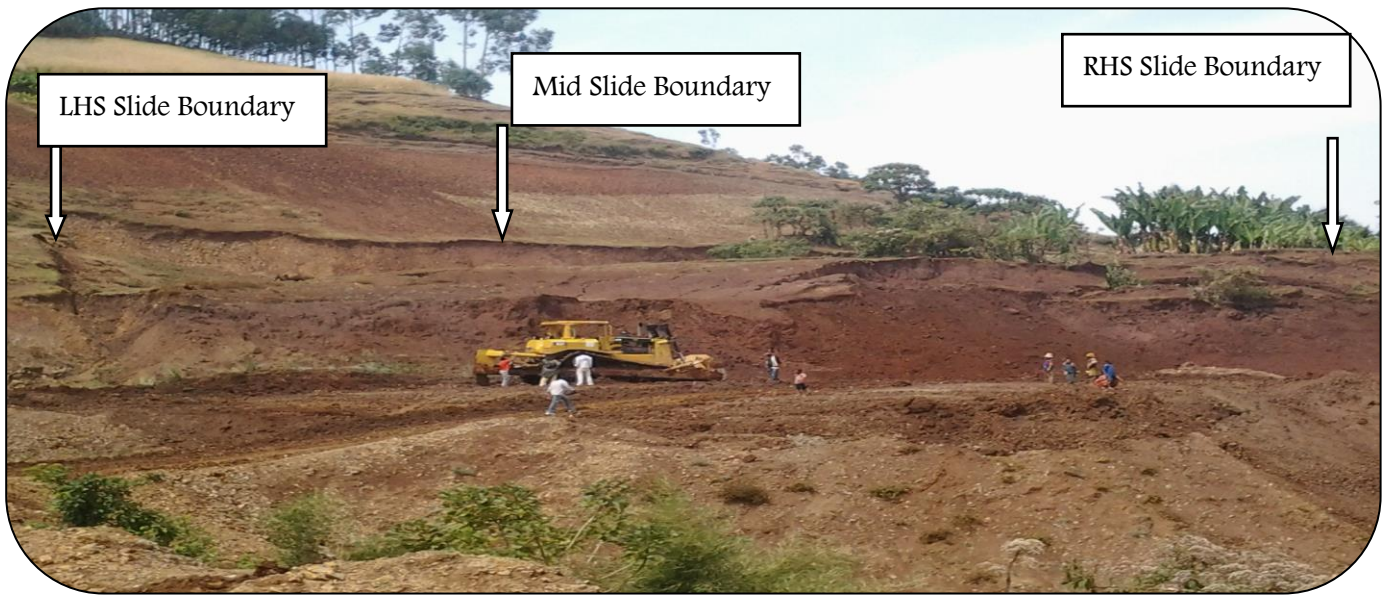
Figure 4.2: Front view of the cut slide manifestation
