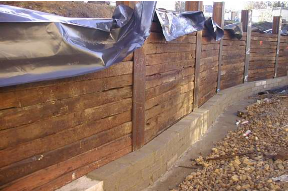
Figure 1. Timber sheet pile wall (source:wikiwand.com).
