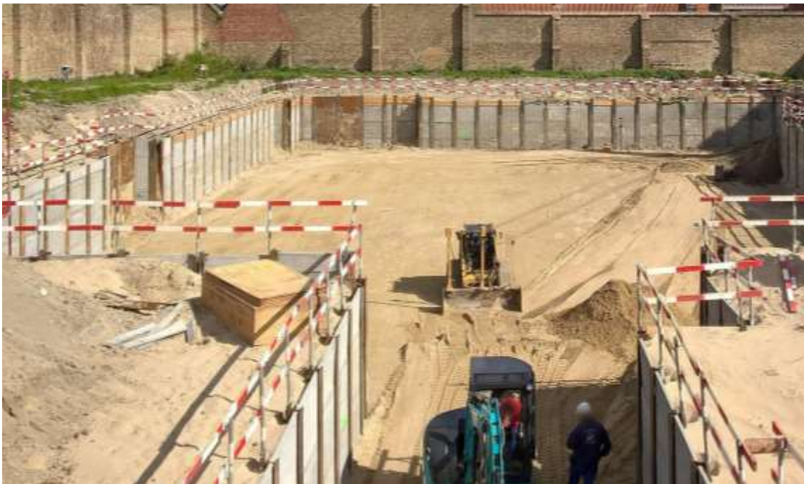
Figure 4. Soldier pile wall (source:theconstructor.org).
