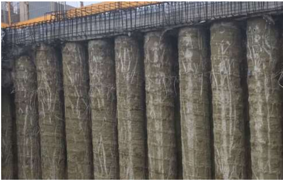
Figure 5. Contiguous piled wall (source:martellopiling.com).
