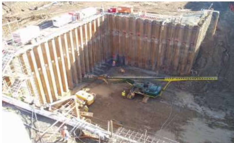
Figure 3. Steel sheet pile wall (source:civilengineeringbible.com).
