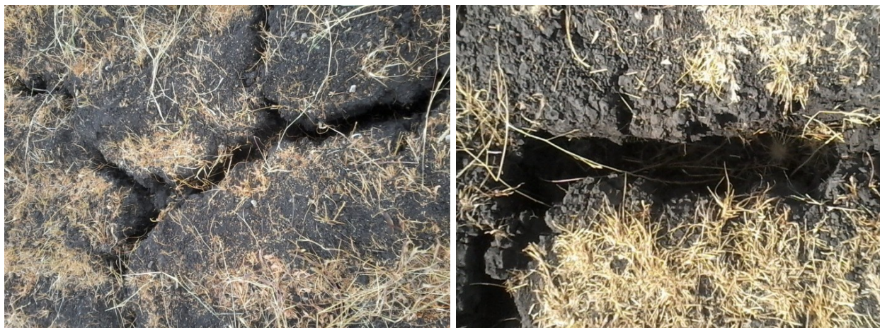
Figure 3.1: visual investigation of crack
