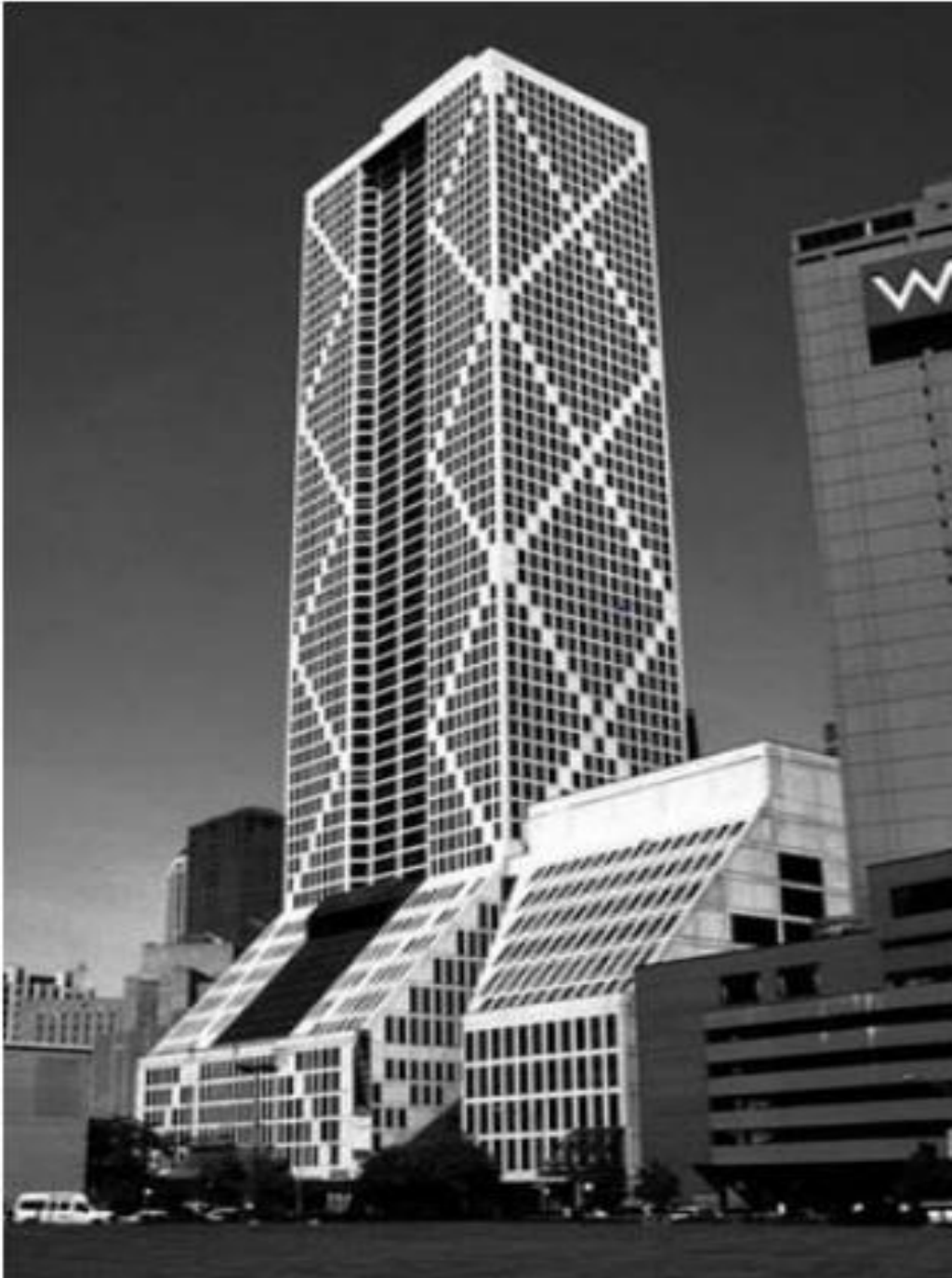
Figure 2-11: Example of exterior diagonal tube: Onyiah Center, Chicago, IL (Taranath, 2010).
