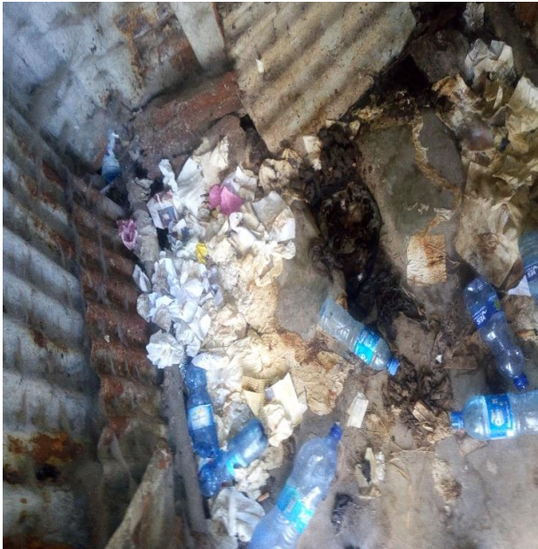
a) public toilets in Kebele 01
