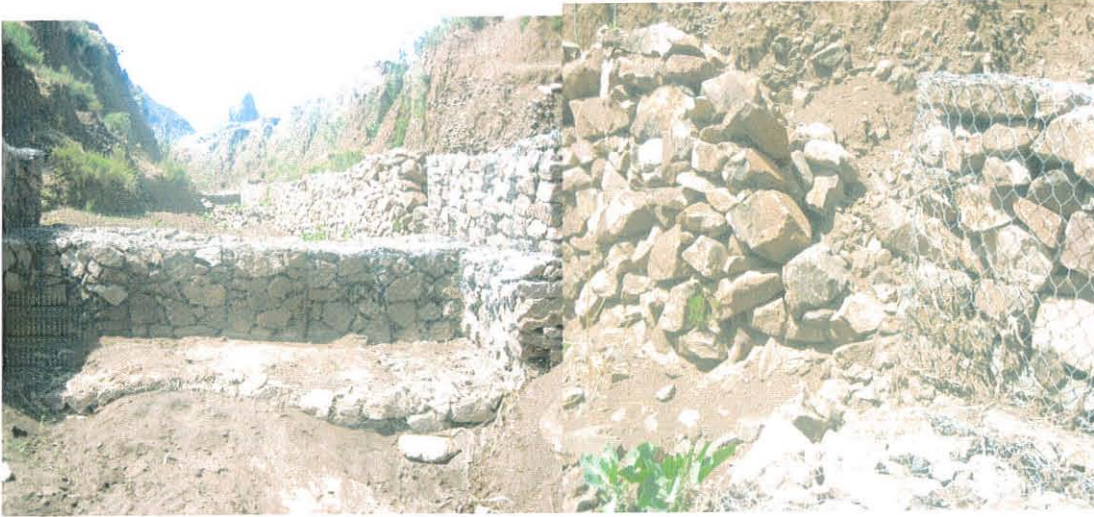
Photo-4.3 Gabions found in good (left) and bad (right) condition.
