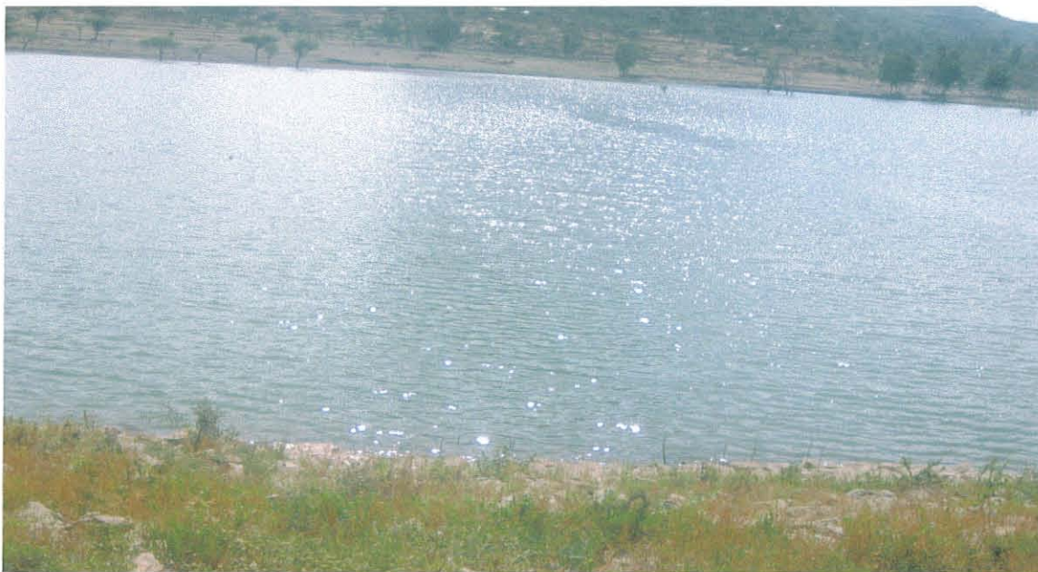
Photo-3.2 Dibdbo Dam
