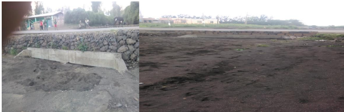
Figure 4-1 Calvert filled by sand
