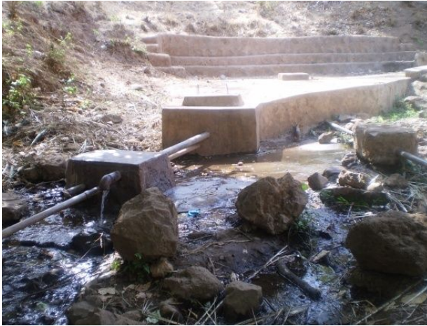
Fig: Spring box and outlets
