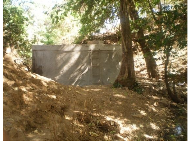
Fig: Storage reservoir
