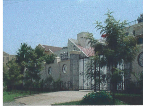
Figure 4.30 Neighboring Rented Residence
