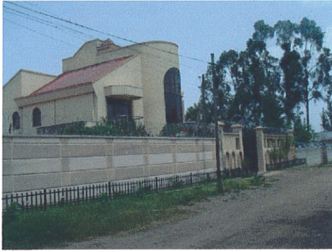
Figure 4.29 Neighboring Rented Residence
