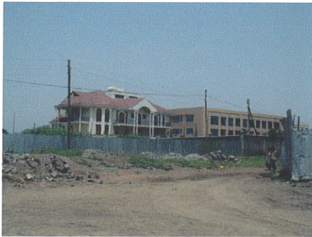
Figure 4.41 Office converted to Luxurious Residence
