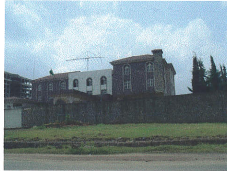
Figure 4.17 Algeria Embassy Chancery.
