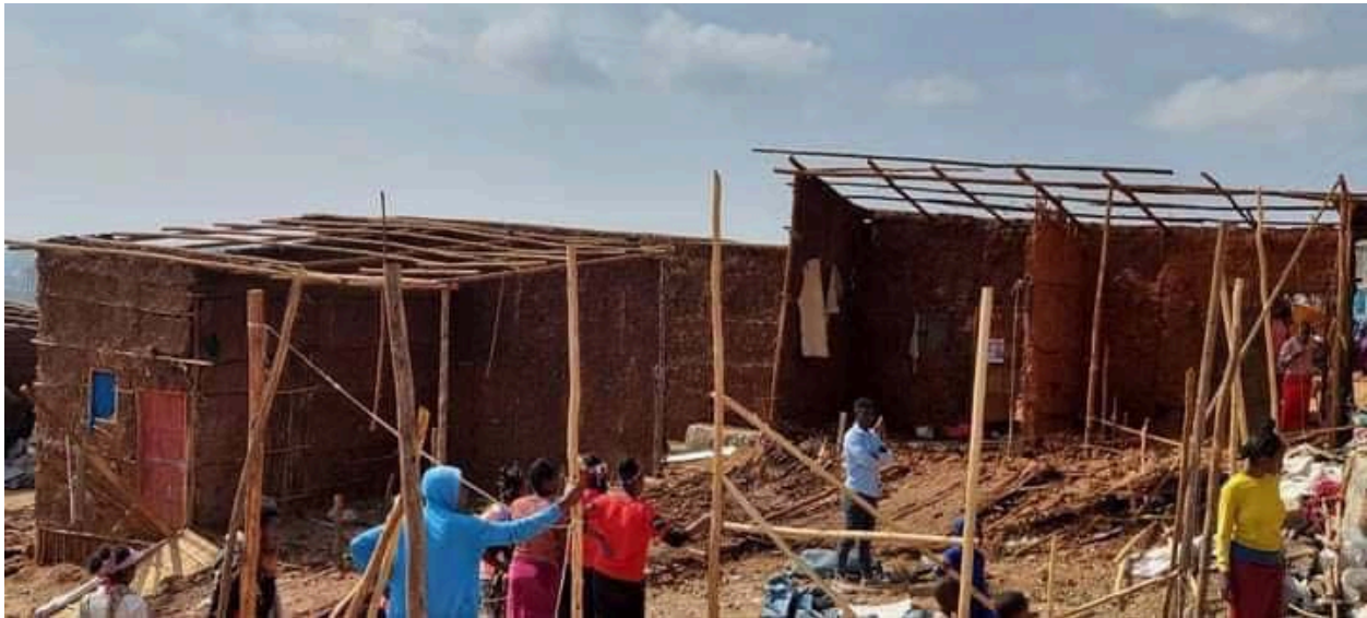
Figure 4 Demolish Campaign near Suke Maryame.
