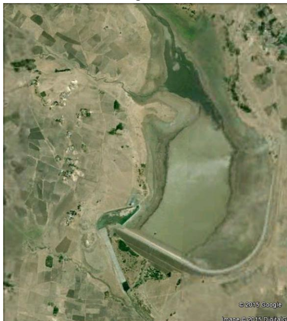
Figure 3-1: Dire impounding reservoir
