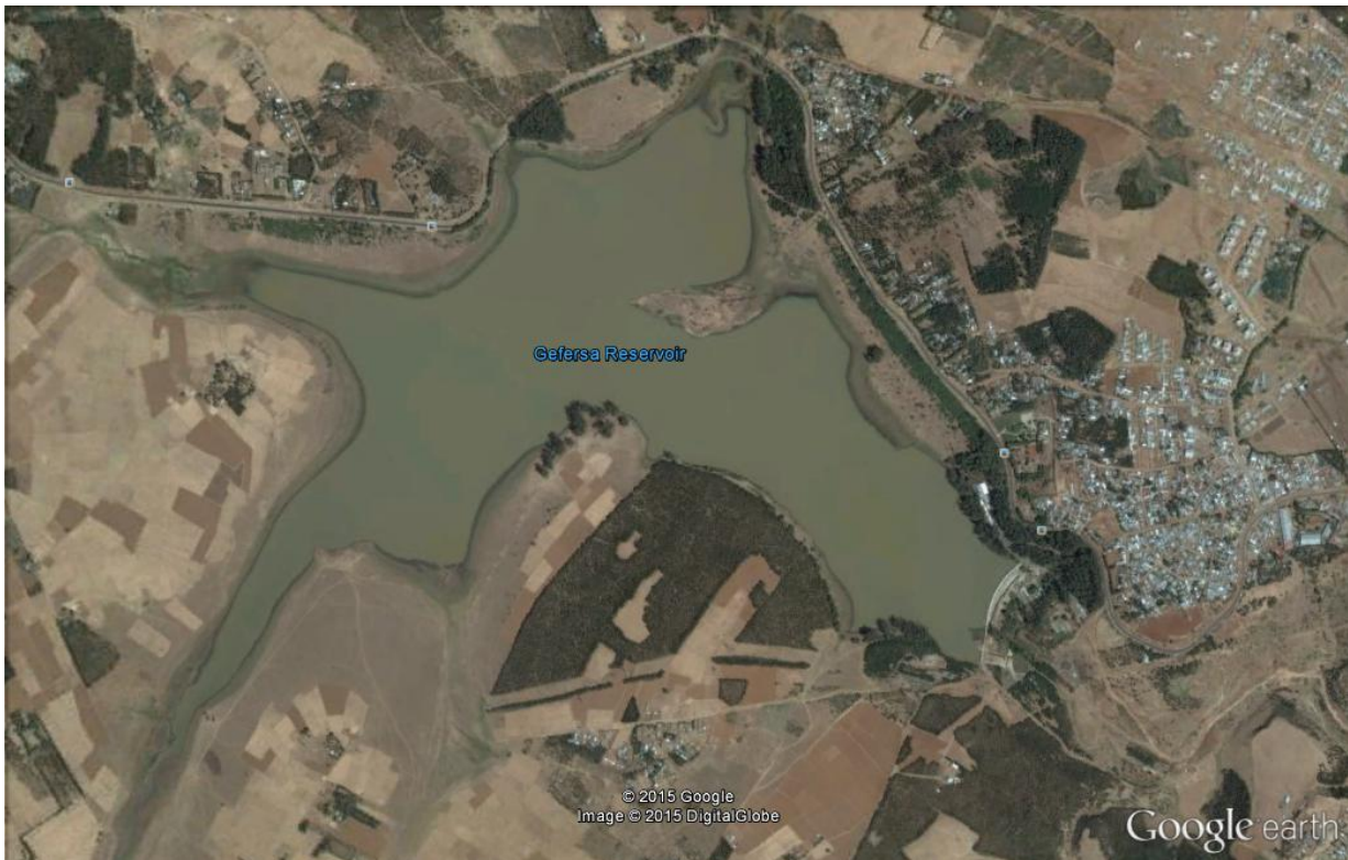
Figure 3-6: Gafarsa impounding reservoir
