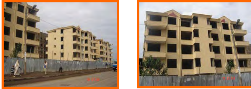
Fig. 134. Photo showing better architectural quality of Sunshine condominiums.
