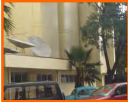
Fig.149. Photo showing a proper place for dish antenna
