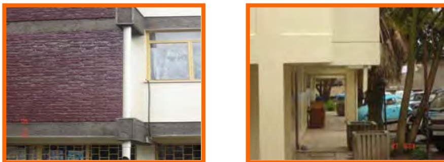
Fig.138. Photo showing material and textures of government rental apartments.
