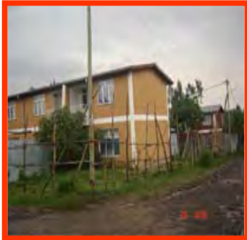
Fig.71. Lack of aesthetics
