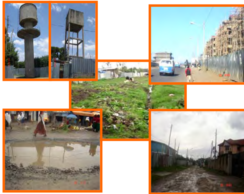
Fig. 132. Photo showing the condition of infrastructure in the case study area
