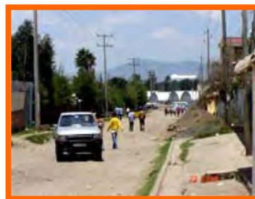
Fig.115Improper floor scape Source:-Field Data, 2007
