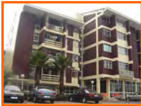
Fig.144. Photo showing the absence of external staircase
