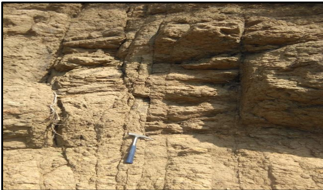
Fig.4.4: Field photograph of unwelded tuff unit with its characteristic unconsolidated and friable nature. Note also the systematic joints affecting it (0561650E:1417549N).
