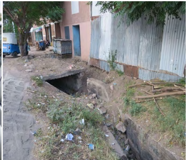
Photo 10: Side drain connection between Municipality & Nazerete-Assela Road Project (Left)
