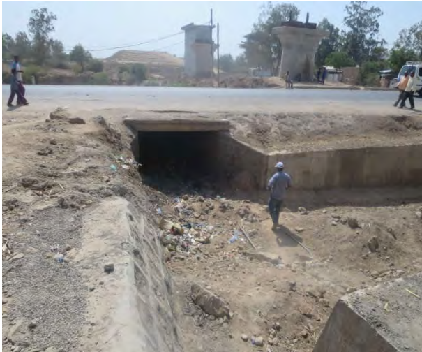
Photo 7: Slab Culvert (Culvert 4) at Km 4+325 (Right)
