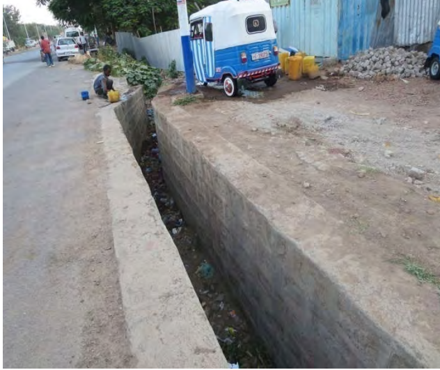
Photo 11: Side drain constructed by the Municipality
