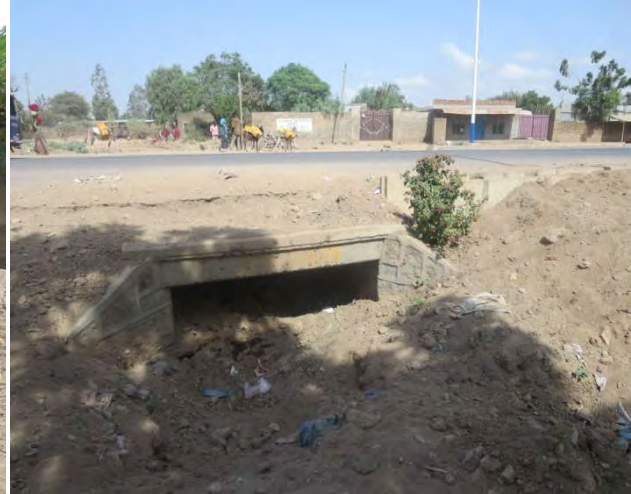
Photo 5: Slab Culvert (Culvert 3) at Km 3+285 (Right)
