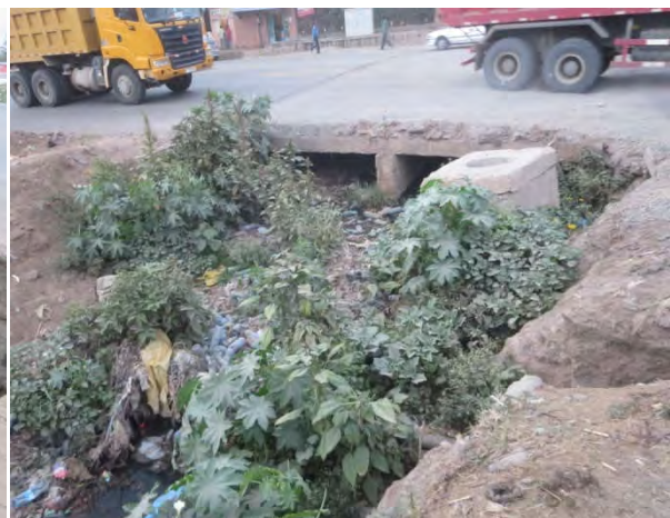
Photo 2: The newly constructed box culvert at the downstream (Left)
