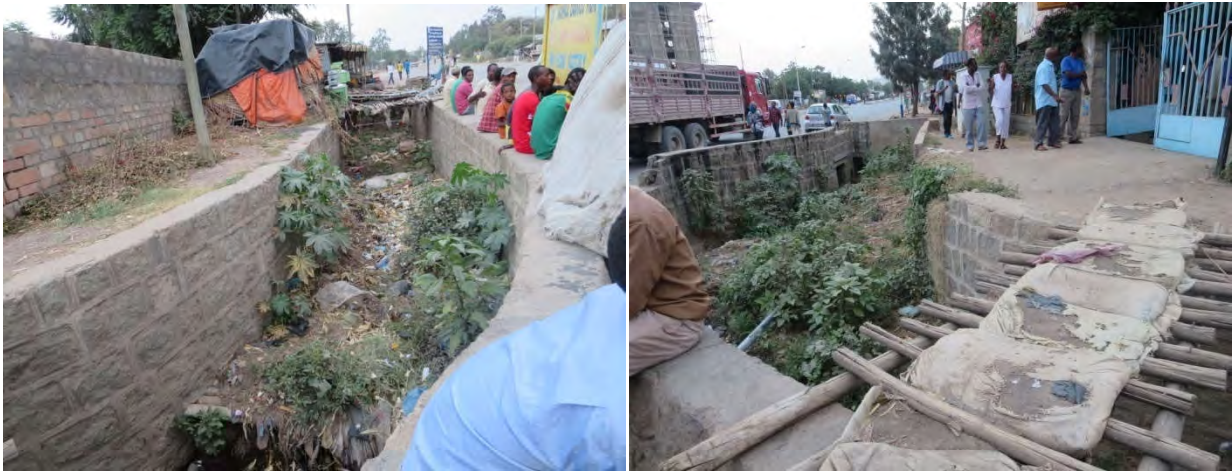
Photo 3: Side drains that discharges at the structures located around Km 2+210
