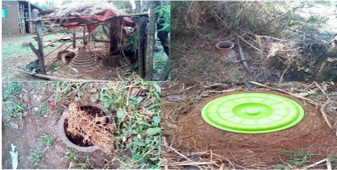
Figure 6: Household Liquid Waste Disposal Facility
