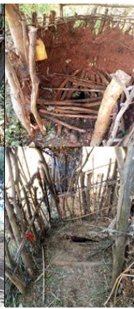
Figure 3-B: Nonfunctional latrine
