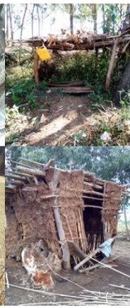
Figure 3-B: Nonfunctional latrine
