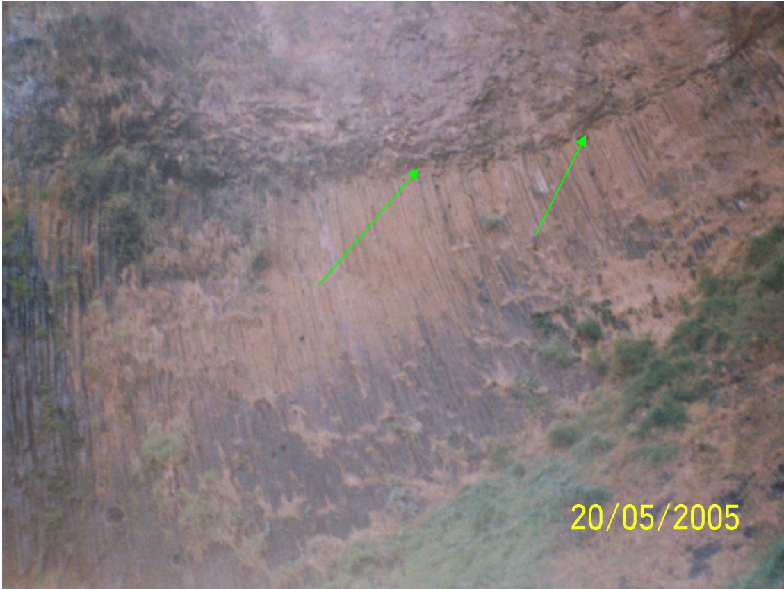
Plate 4 .5 contact between over-ling rhyolite and under-lying fresh basalt
