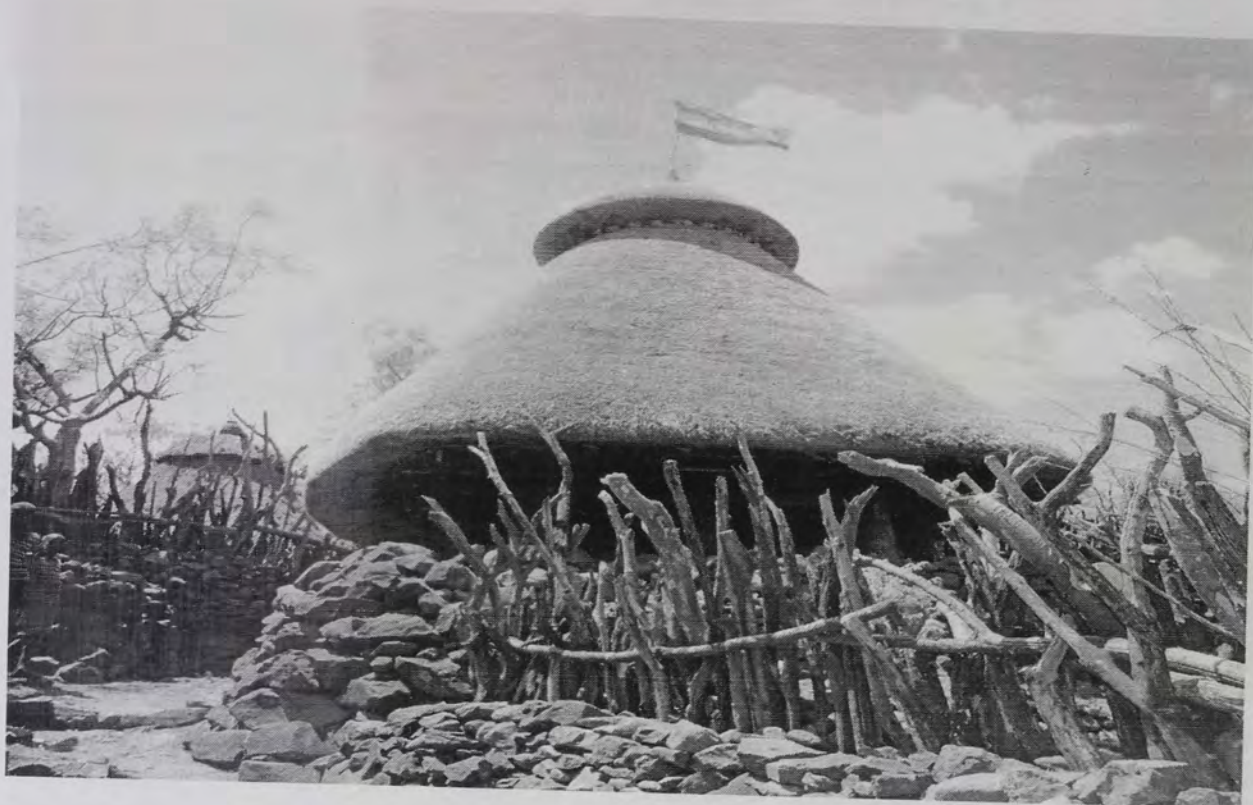
Plate 12. The newly built thatched house on Moora Lehaytii in the Dekatto Alaka with the Ethiopian flag
