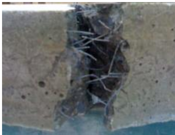
Fig.4.9 Sample beam failed by fibre pullout under flexure
