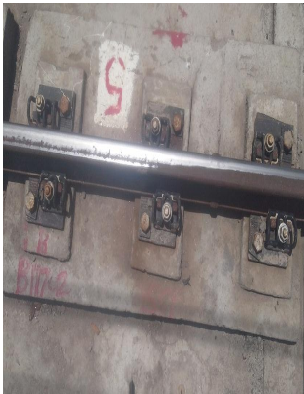
Fig.1.1 Bridge slab sleeper around Legehar
