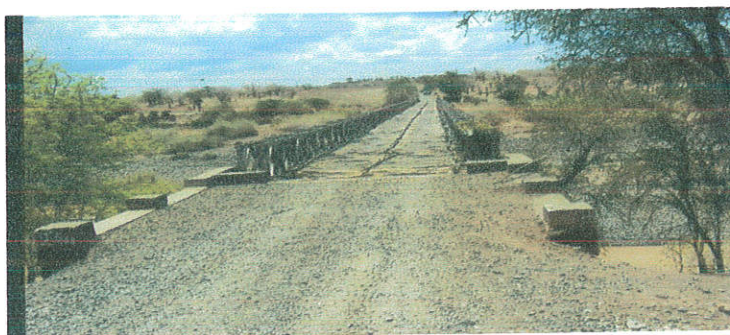
Photograph 21 and 22: Overhead view and side view of the Angäräb Bailey Bridge
