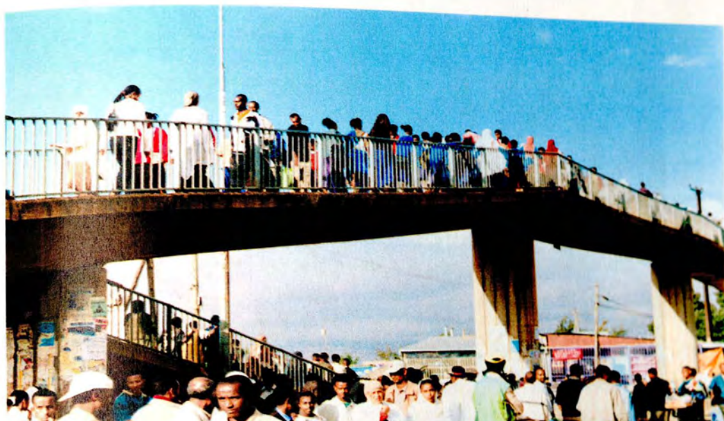
Plate3: Pedestrians crossing the highway
