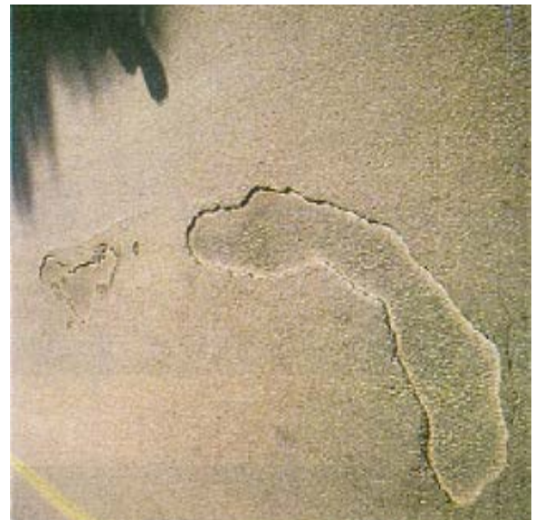
Plate 2.8 Stripping in Asphalt
