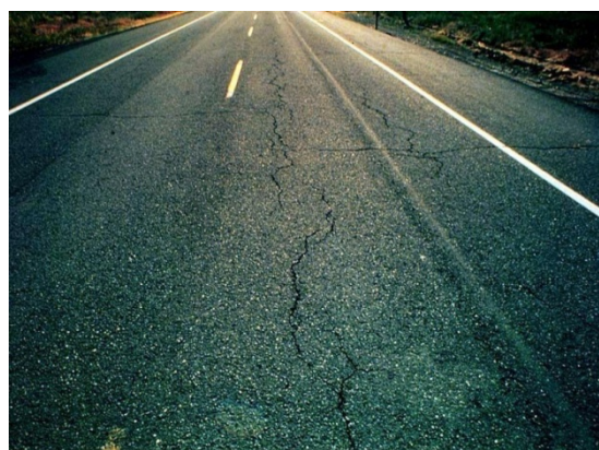
Plate 2.3 Longitudinal Cracking
