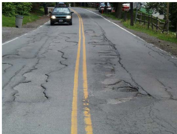
Plate 2.17 Delamination
