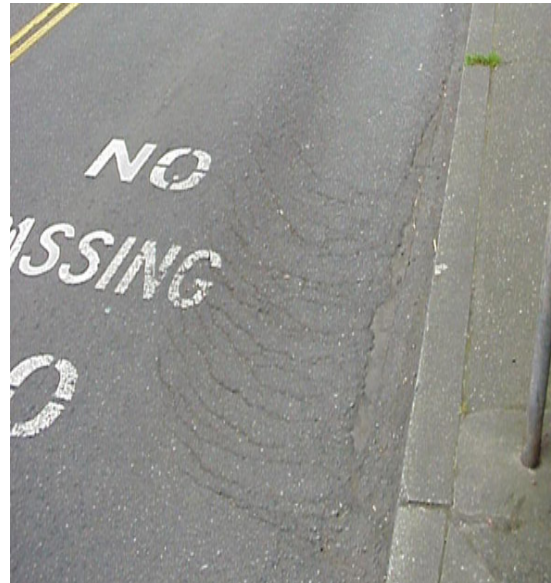
Plate 2.14 Slippage crack
