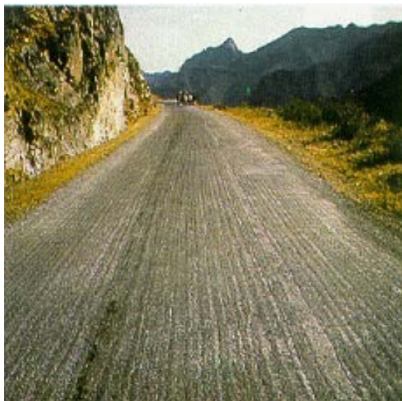
Plate 2.7 Fretting of aggregates
